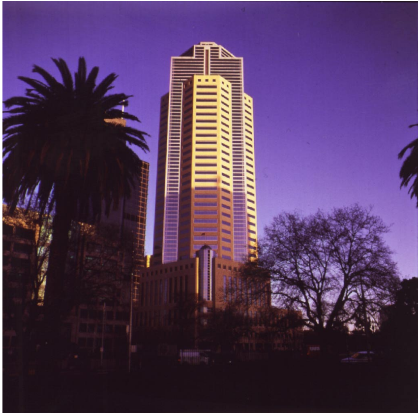
Casselden Place, Melbourne, Australia
